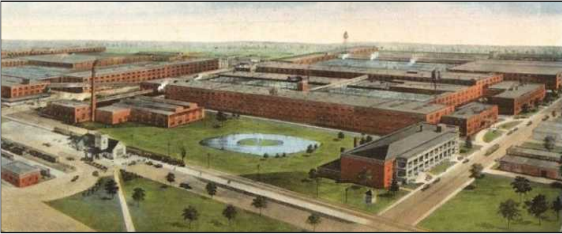
THE REO Motor Car Co. works in Lansing, in a circa 1920 postcard. Closed in 1975, many of the still-intact buildings were placed on the National Historic Register in 1978. Then they were demolished in 1980. Today commercial buildings populate the site.
