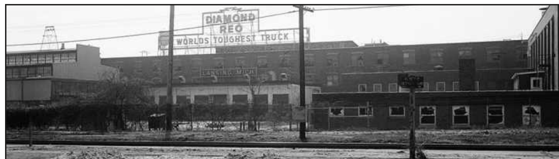
THE REO MOTOR WORKS factory was built in 1905, and is shown here in 1977 awaiting demolition. Photo credit: National Parks Service/Ralph J. Christian
