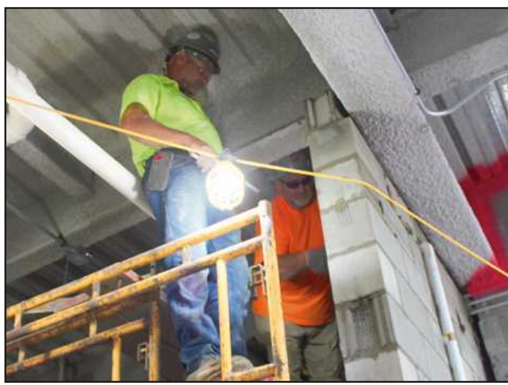
SETTING A BLOCK WALL inside the Saginaw United High School building are (l-r) Daryl Labean and Jack Fenton of Bricklayers and Allied Craftworkers Local 2. They're employed by Davenport Masonry.
