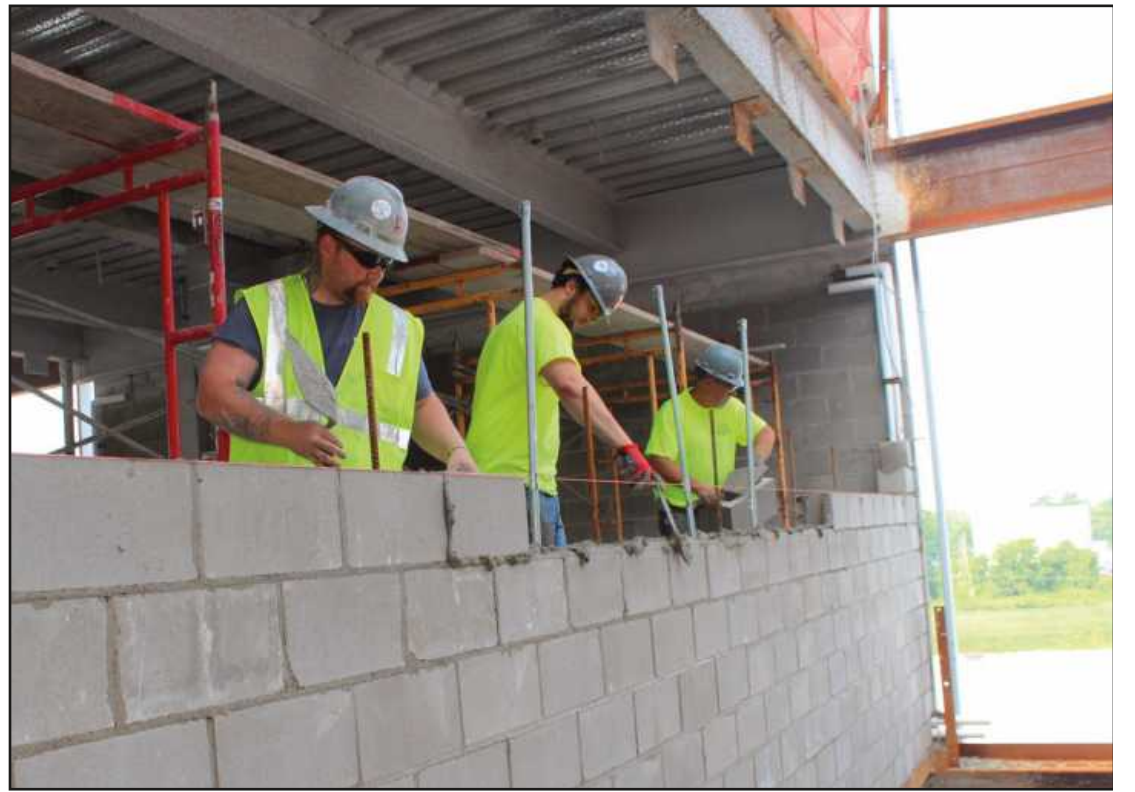
LAYING A COURSE OF BLOCK at the Saginaw United High School project are Troy Jacobs, Eric Bootz and Nathan Taljonik of Bricklayers and Allied Craftworkers Local 2. They're employed by Davenport Masonry.
